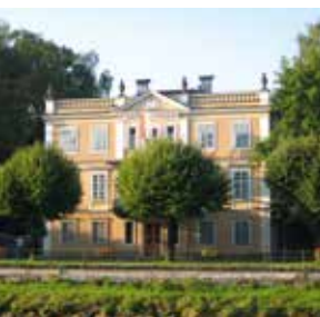
The Lehar Villa: the master composed thirty of his works here.
