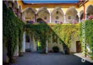
Visible for miles around, the Körblerhaus is among the best-preserved and most beautifully renovated town houses in Judenburg's main square.
