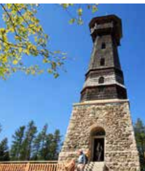
Ringwarte, historical lookout post on the Ringkogel, which was colonised long ago by the Celts.
